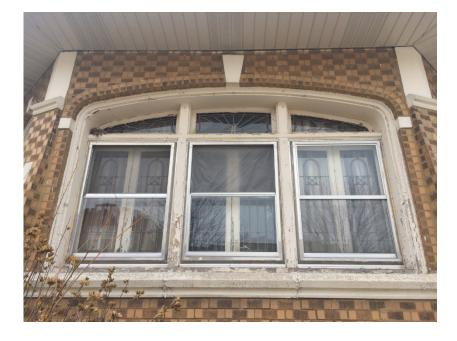
Old wood windows are a common source of lead hazards, along with doors and door frames, stairs, and porches.
